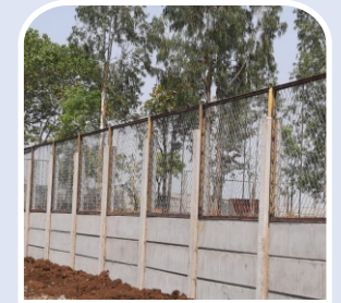
LAYOUT FENCING & DEMARCATION
